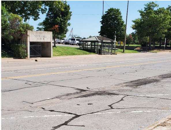
Downtown Transfer Center
